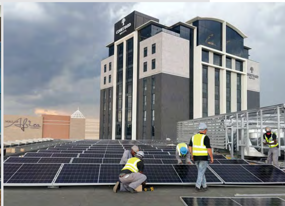
Installing a 230kWp rooftop PV system on Nexus Waterfall - building 1, Waterfall City
