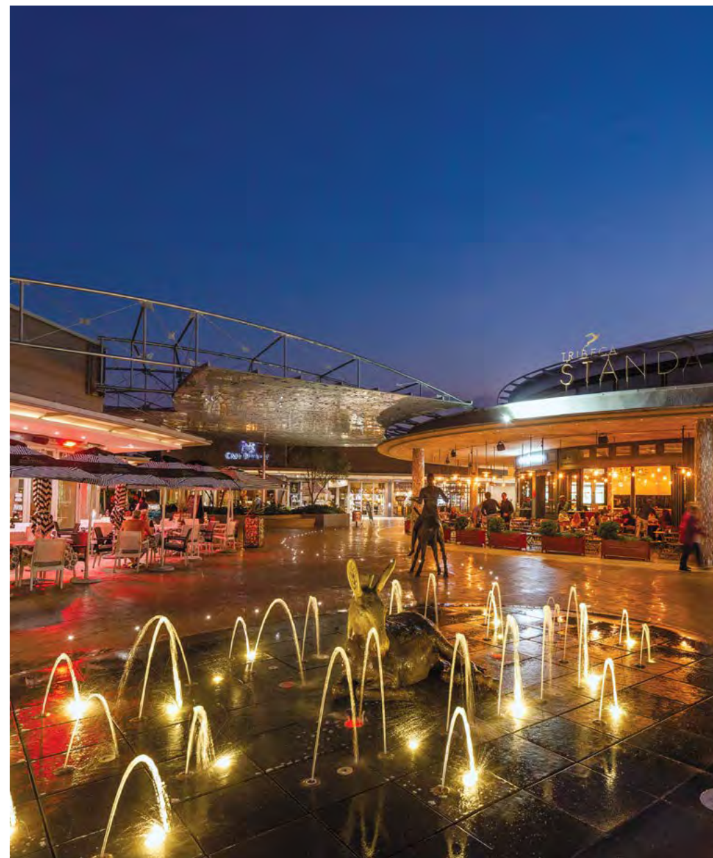
Lynnwood Bridge precinct - retail, Pretoria
